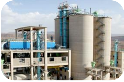
Construction Materials Industry
