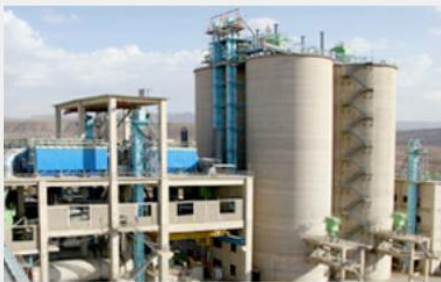
Construction Materials Industry
